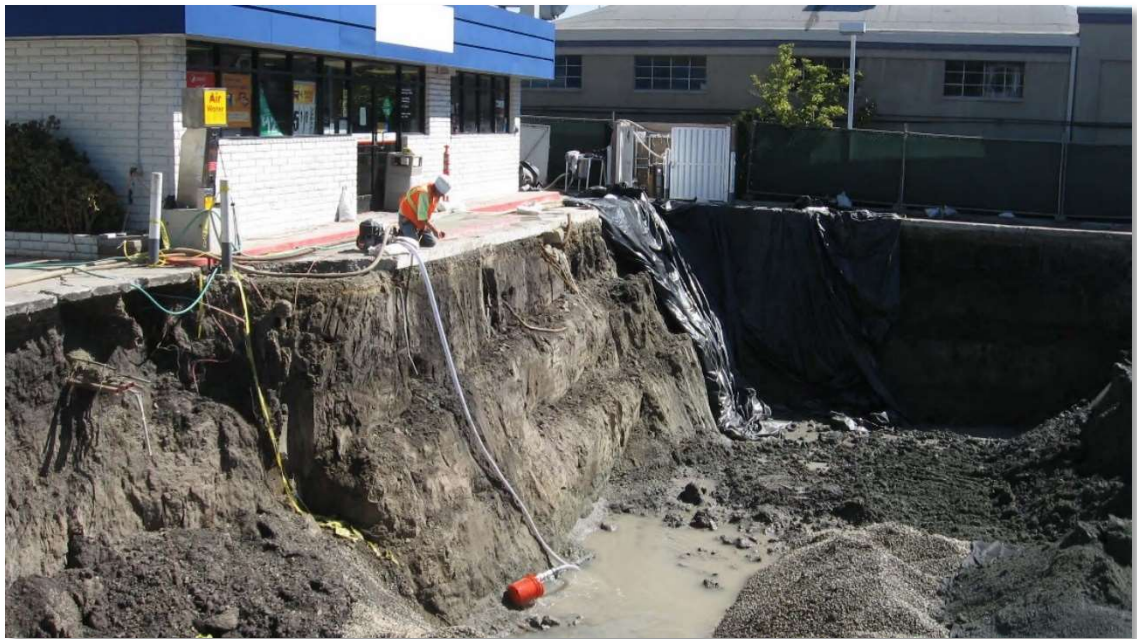
26 Defendants’ Partial Excavation of Contaminated Soil from Leaking USTs, circa 2012
